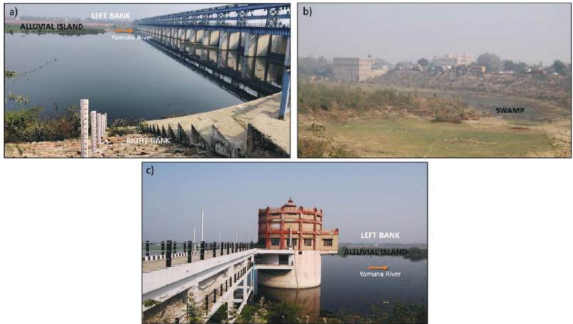
Figure 131: (a) U/S of Gokul Barrage. Alluvial Island can be observed; (b) Swampy/Marshy area in the proximity of the Barrage; (c) Intake well.
